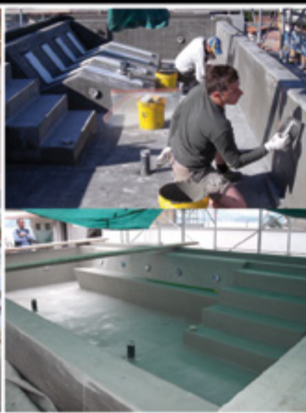
○ Laying, levelling and waterproofing
