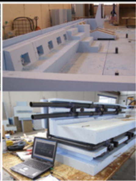
○ Manufacturing of structures in EPS and on-site installation of equipment
