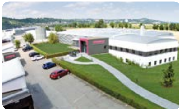
The current company buildings have been refurbished for energy and are invitingly laid out
