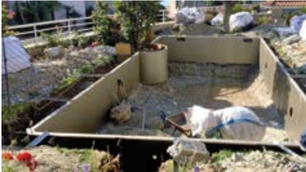
Installation de la structure
