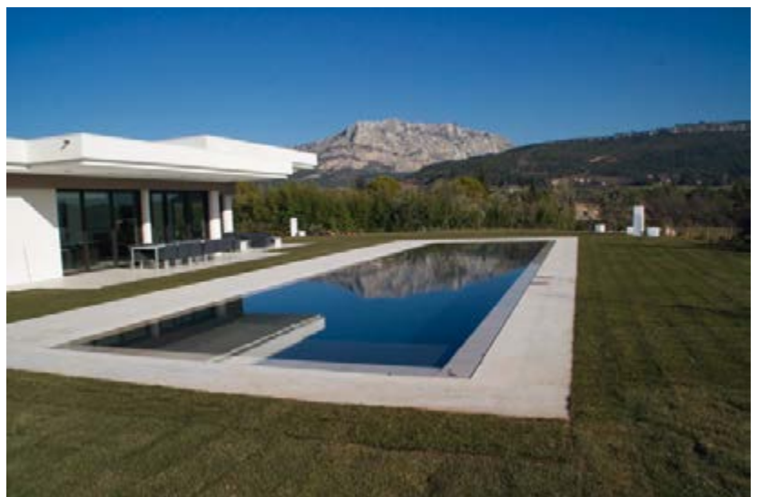
Piscine béton procédé Leader Pool, miroir, 20 m x 5 m, carrelé (MGA Concept - 13)
